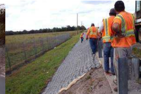
Side Slope Improvements
