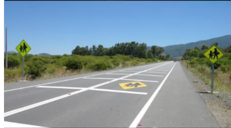
Speed hump (up), Transverse lines on both lanes (down) (Source: PIARC, 2019)
