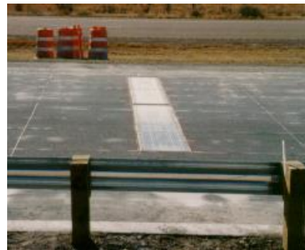
Figure 2: Bending plate detail
