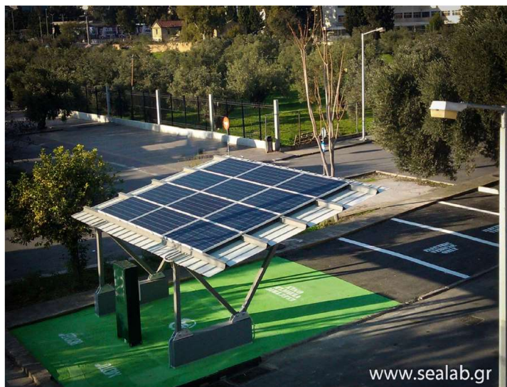
Figure 4: Charging station developed and installed by the SEALAB of the Piraeus University of Applied Sciences (Kaldellis et al., 2015)
