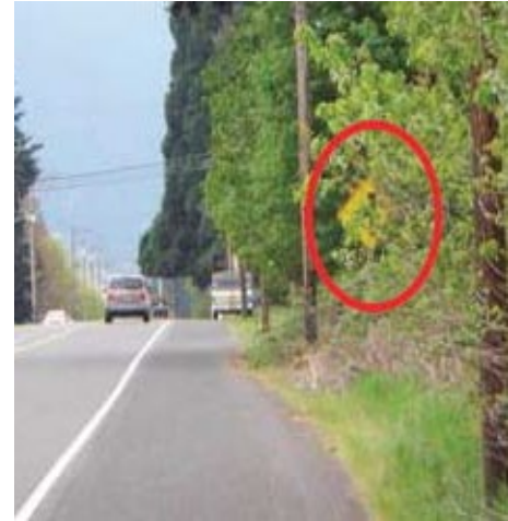
Figure 2: Sign Occluded by Vegetation (Image source: FWHA)
