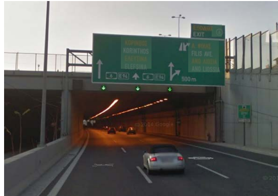
Figure 3: Tunnel entrance-conditions of high workload (image from google maps)
