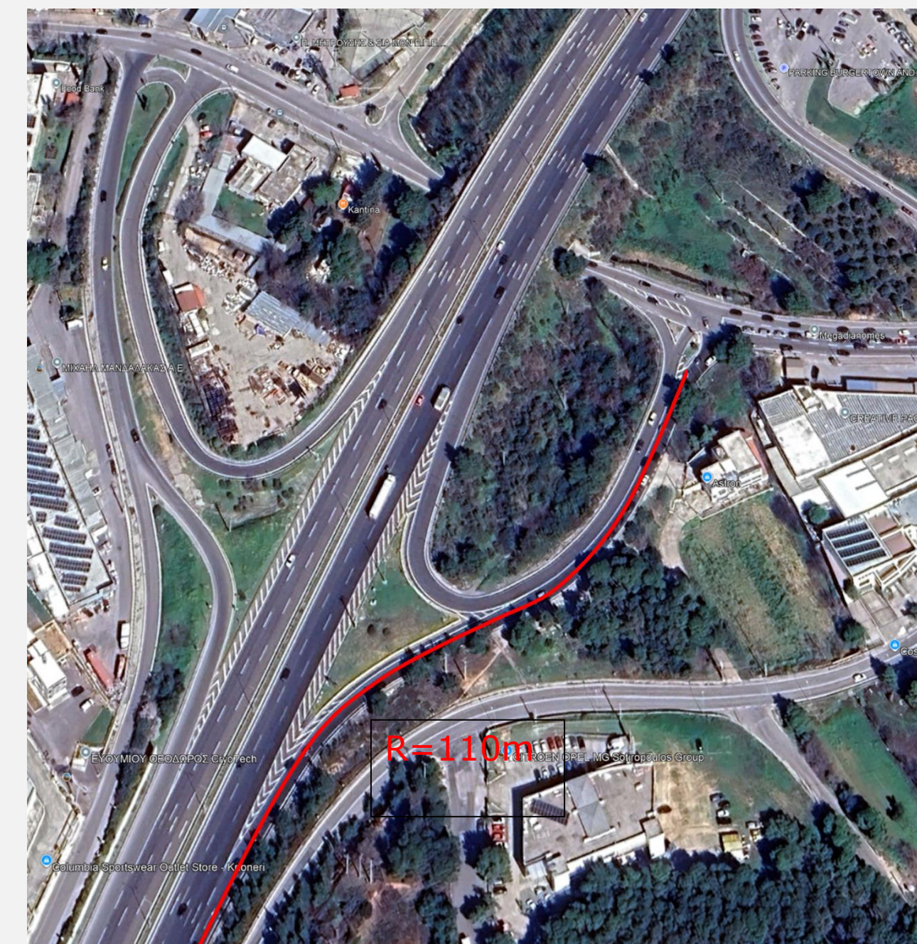
Semi-directional exit ramp of Agios Stefanos IC
